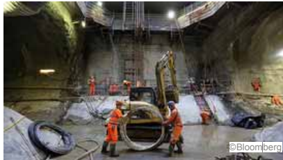
A Crossrail construction site at Stepney Green in east London
