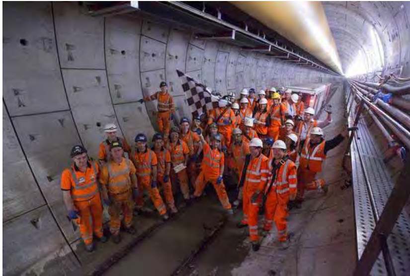
Halfway: Crossrail workers celebrate as 13 of the 26 miles of tunnel are completed
