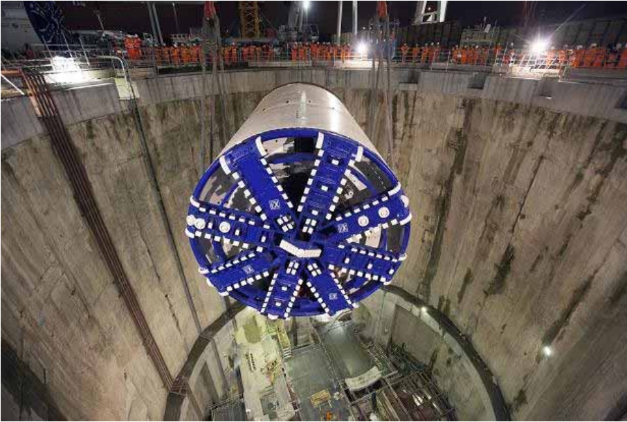
The trains for Crossrail, still under construction, will run from east of Whitechapel to Paddington EFA/Crossrail
