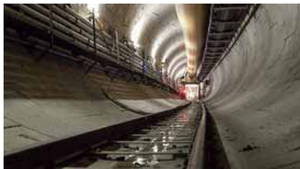
Tunnels under construction for the Crossrail route
