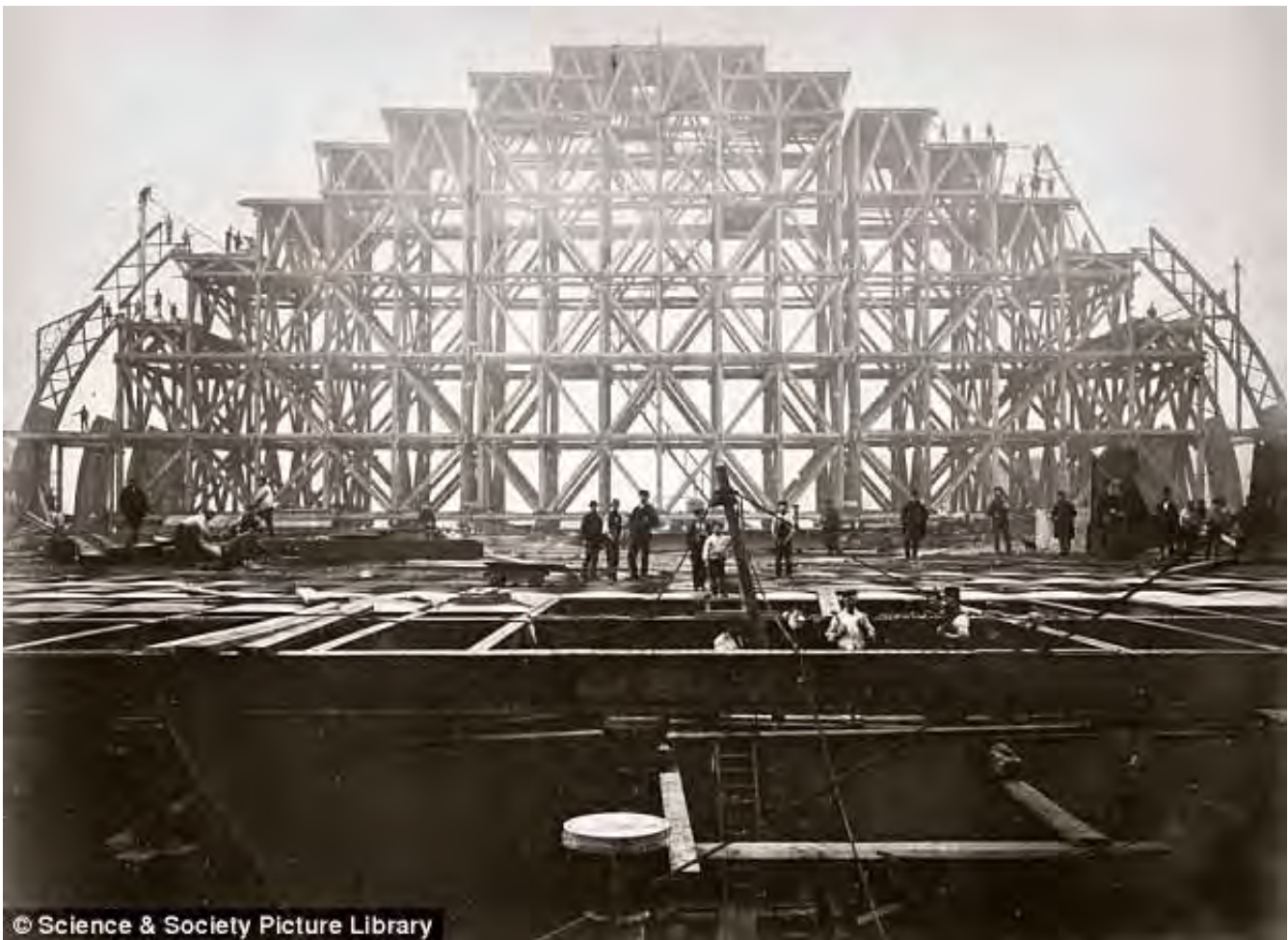
Construction: Butterley's went into administration in 2009 but provided the ironwork for some of Britain's most iconic buildings, including Vauxhall Bridge and the roof of St Pancras station (pictured here in the 1860s)
