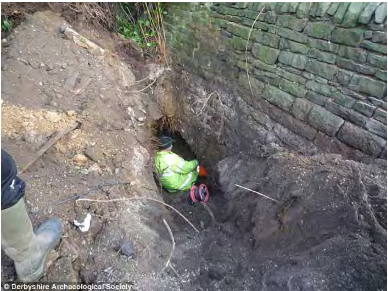
Lost: The tunnel was sealed up 1977 by a previous land owner to build a rockery. The dig began in January and used heavy machinery to re-open the sealed passage
