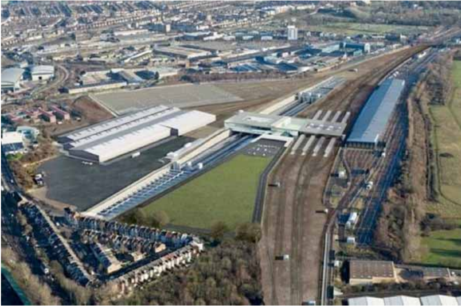
How it could look - Old Oak Common with Crossrail depot plus Crossrail/HS2 interchange station
