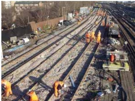
A second 54 hour possession in November saw the same process used to install the other switch as well as the crossover into the Down line. The crossover was connected to the Up line switch installed previously. Both possessions went to plan, and the line was handed back on time and with no delays.
