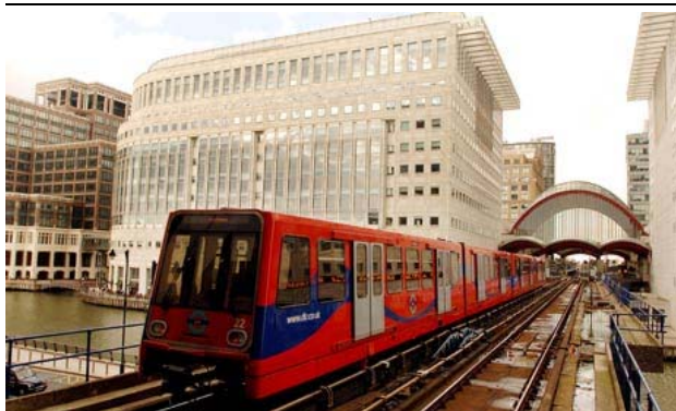
The Docklands light railway in east London. Photograph: John Stillwell/PA Archive/Press Association Ima
